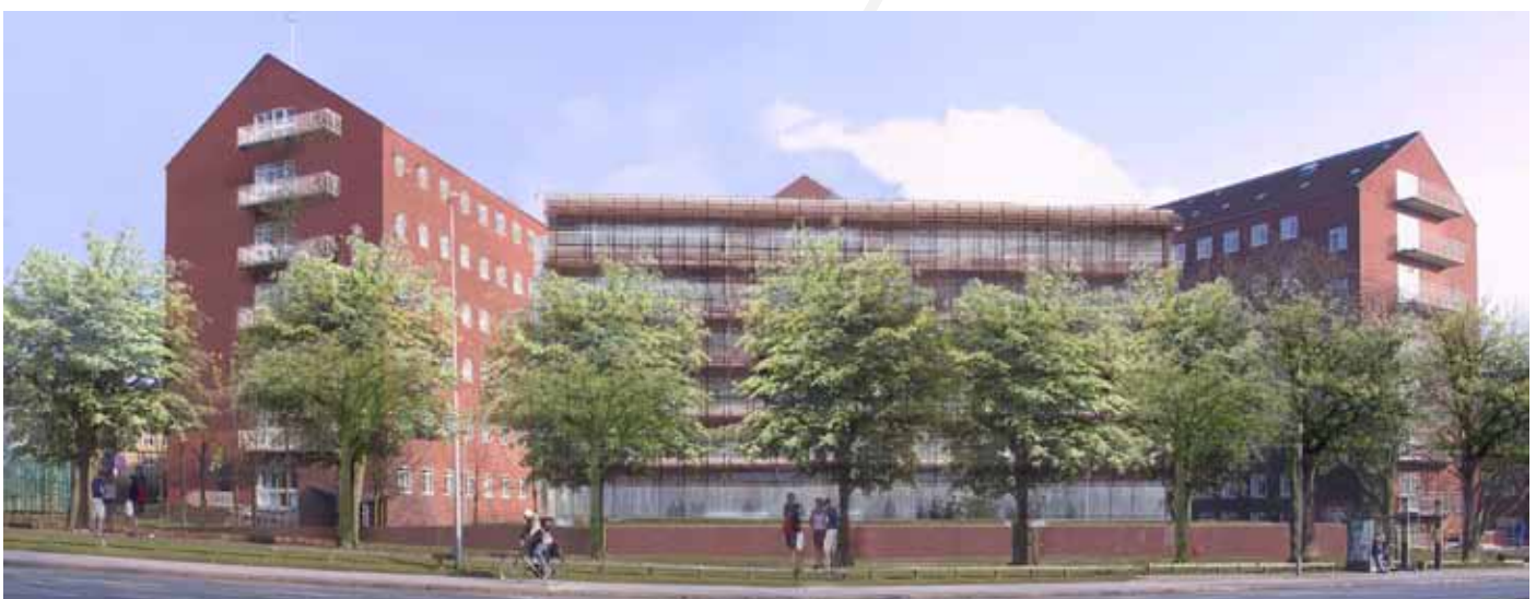
DNC Building facade to Nørrebrogade - Architect company C. F. Møller
